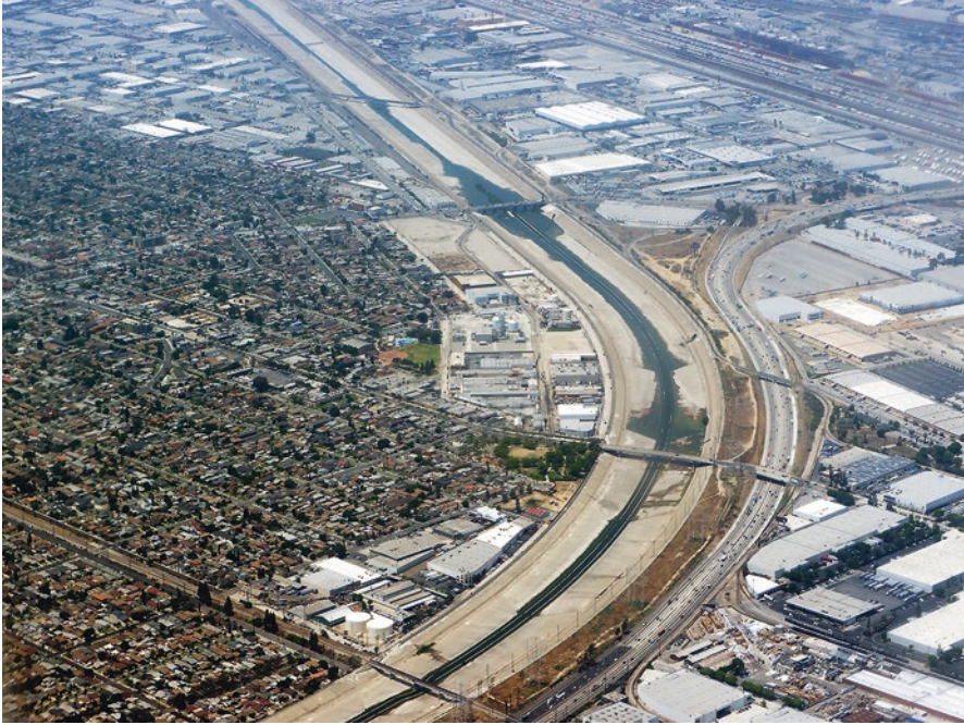
Fig. 3.6 Channelizing the Los Angeles River. After devastating floods in 1934 and 1938, the US federal government embarked on a massive flood control program in Los Angeles in the 1950s, straightening and channelizing the Los Angeles River with 3.5 million barrels of cement and 147 million pounds of steel. With concrete lining its banks for 94% of its course, the river, once the lifeblood of the city, became a “fifty-one-mile storm drain.” (Source: Image courtesy of Brian C. O’Connor, 2014)
