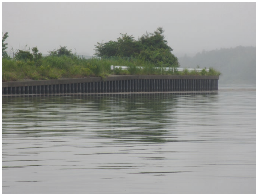
Fig. 28.4 Today more than 80% of Kamoko's shore is covered by pile-sheet revetment. (Photo Mitsuyo Toyoda)
