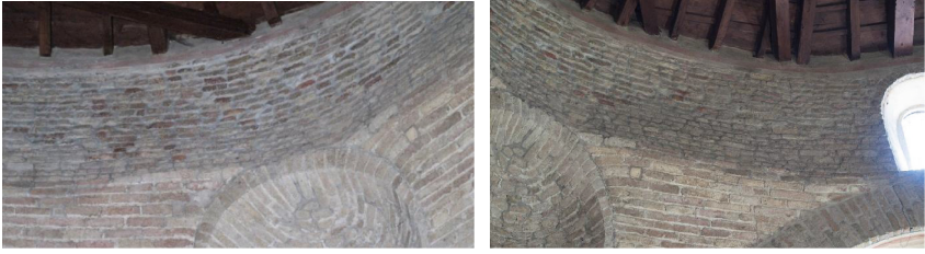
Fig. 2. Detail of the drum masonry pattern
