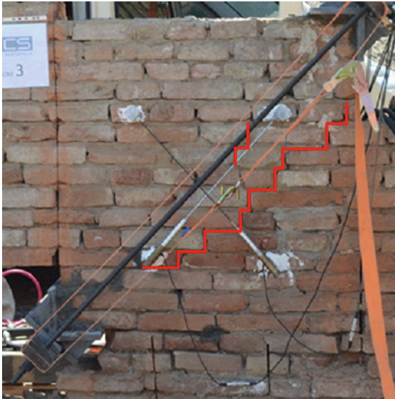
Fig. 1. Typical crack pattern obtained at failure in unreinforced panels.
