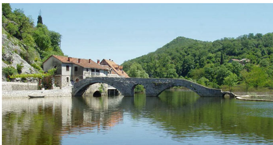
Fig. 9 The old bridge called “Mostina” in Rijeka Crnojevića. Photo by D. Dajković
