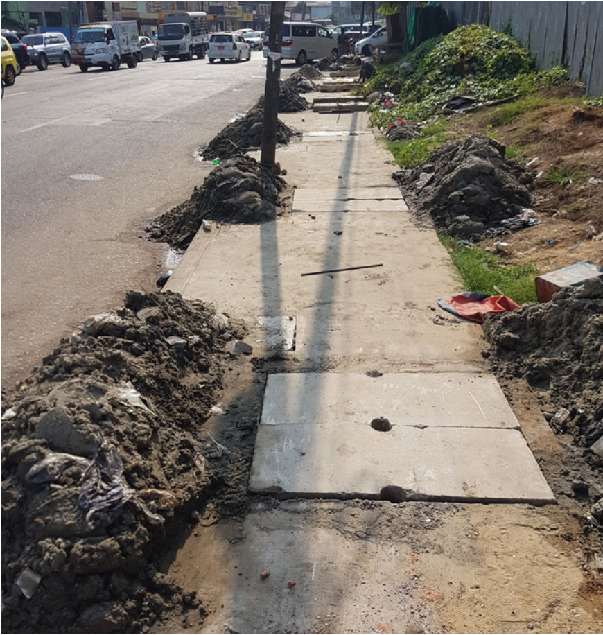
Fig. 6.5 Drainage canal being dredged by hand (Photo by Graham Reeder)
