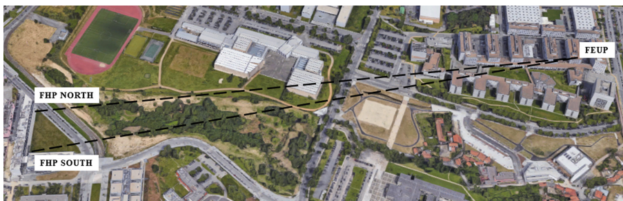
Fig. 4. SV4D testbed installation in Porto, Portugal.
