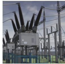
Fig. 2. 3D model of a 110 kV SF6 circuit-breaker.
