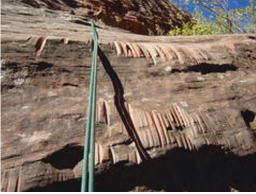
Fig. 4.4 Rope damage to Sandstone, Zion National Park, Utah. Photo by D. Huddart
