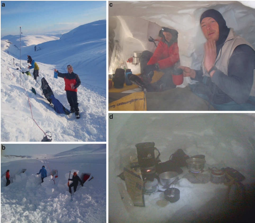
Fig. 8.3 (A) Excavating snow caves at Garbh Uist Beag, Cairngorms, Scotland. Photo by Tim Stott. (B) A snow cave is constructed by excavating snow so that the tunnel entrance is below the main space to retain warm air. Photo
