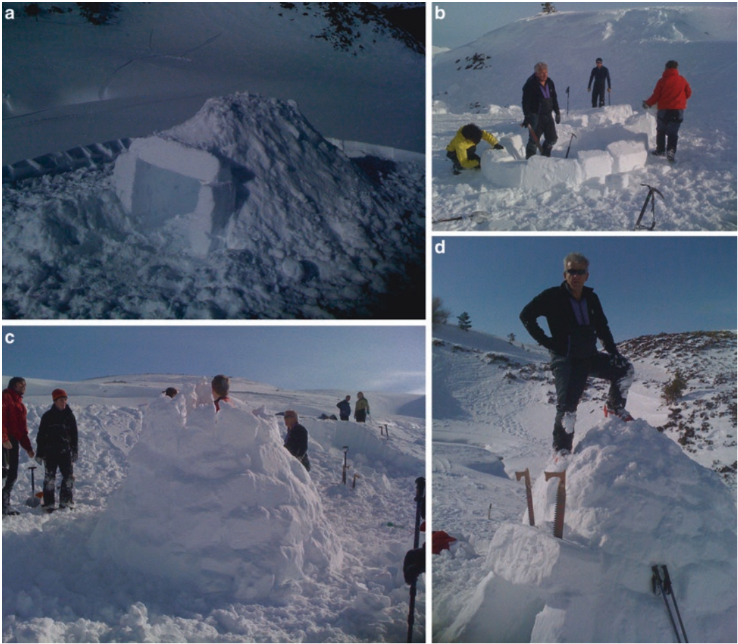
Fig. 8.4 (A) A quinzhee (or quinzee) is a snow shelter that is made from a large pile of loose snow which is shaped then hollowed. Photo by Tim Stott. (B) Cutting snow blocks to make the base of an igloo, Cairngorms, Scotland.
