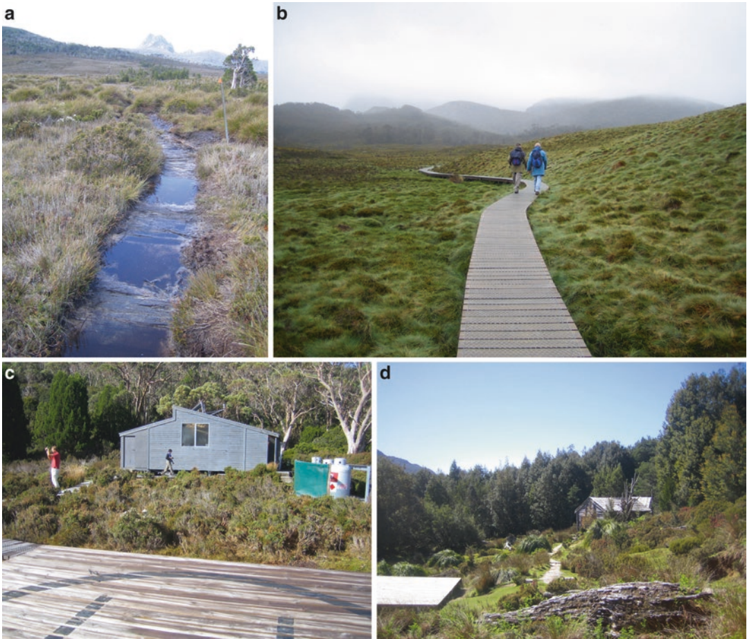
Fig. 8.9 (A) A degraded section of the Tasmanian Overland Track (2005). Photo by Tim Stott. (B) A renovated section of the Tasmanian Overland Track (2005). Photo by Tim Stott. (C) Hardening of campsites at selected overnight nodes (foreground) on the Tasmanian Overland Track com-
