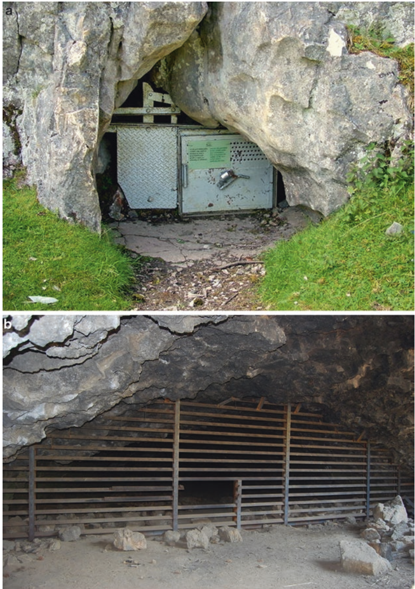
Fig. 12.6 (A) Gating at Agen Allwedd, Llangattock, South Wales. Photo by D. Huddart. (B) Bat Gate at the entrance of Skeleton Cave, near Bend, Deschutes County, Oregon; lava tube on the northern flank of Newberry volcano. Photo by United States Forest Service
