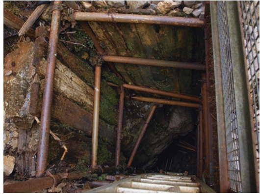
Fig. 12.3 Great Douk dig, vertically from the collapsed cave entrance section to try and connect the active streamway from the cave to the River Greta to the west. Note the shoring, scaffolding, and ladder. Photo by D. Huddart
