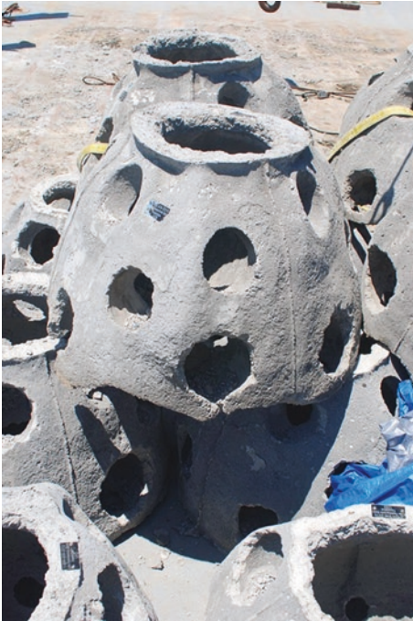
Fig. 14.7 Reef balls, Lake Pontchartrain Basin. Source: Louisiana Sea Grant College Program, Louisiana State University, USA
