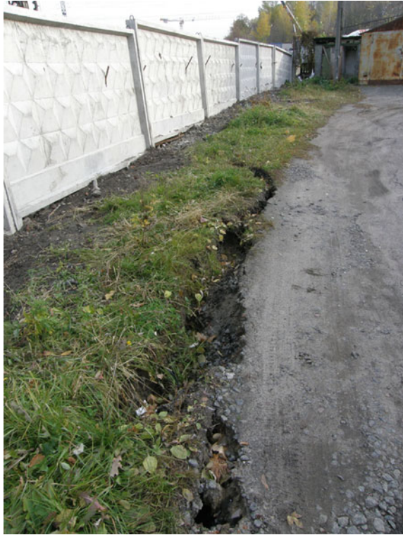
Fig. 31.2 Formation of the landslide zone in the area of Western underground water flow
