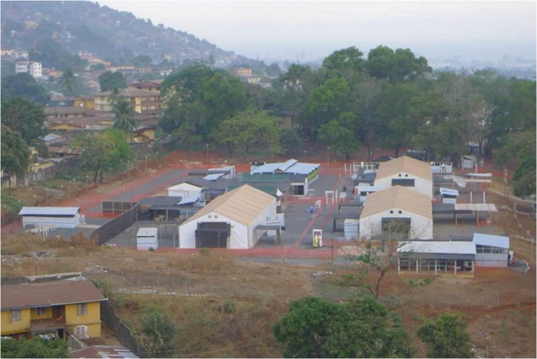
Fig. 20.2 Aerial view of the METC in Kissy, Freetown. Published with permission of © Doctors Without Borders/ Médecins Sans Frontières 2018. All Rights Reserved
