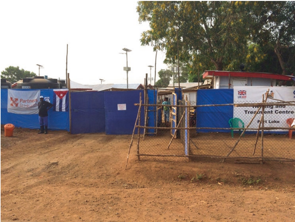
Fig. 5.1 Front entrance of Maforki Ebola Holding and Treatment Centre, Port Loko, Sierra Leone
