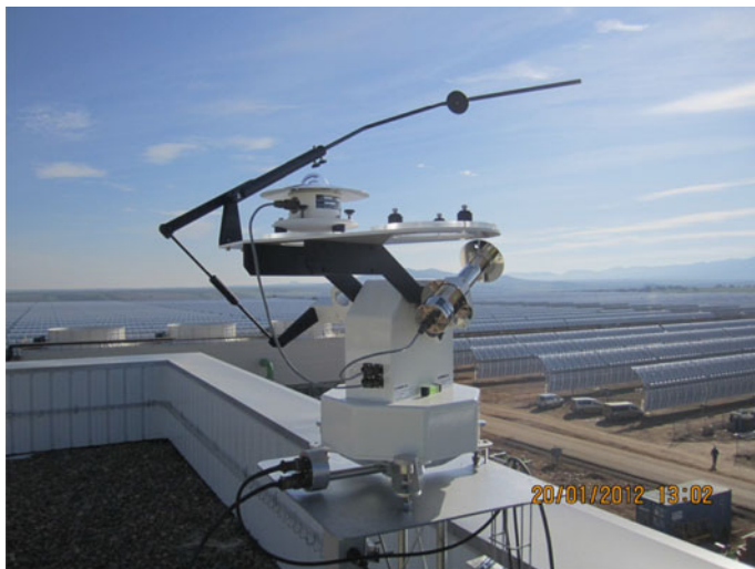
Fig. 20 SunTracker-3000 at concentrated solar power (CSP) plant. Courtesy of Geonica ©
