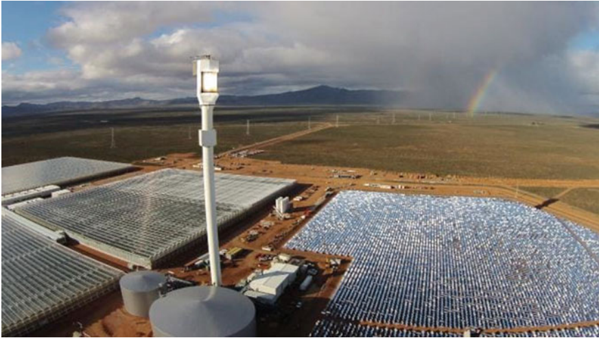
Fig. 7 Overall view of the Sundrop Farms Facility
