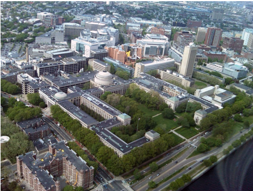
Fig. 27.6 Cambridge, Mass—Innovation District. Aerial view of part of MIT’s main campus. By DrKenneth, Wikimedia Commons, https://commons.wikimedia.org/wiki/File:MIT_Main_Campus_Aerial.jpg
