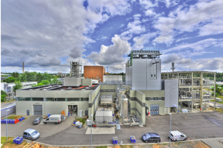
Fig. 6 Image of the bioliq ® pilot plant at KIT. From left to right : fast pyrolysis plant, biosyncrude storage, EF gasifier, gas cleaning section, and synthesis plant in outdoor construction
