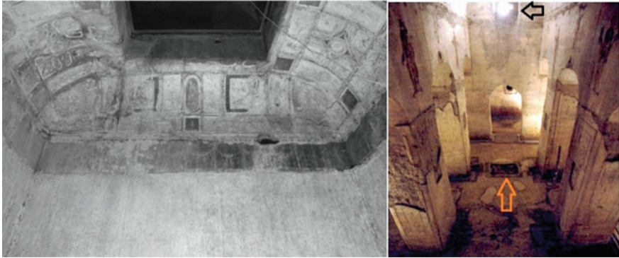
Fig. 4.5 Left: the skylight in the vestibule. Right: The wall between the nave and the vestibule. Notice the hopper window (black arrow) and the imprint of the altar (orange arrow) on the floor between the two first pillars (courtesy: Rome Archaeological Superintendence)
