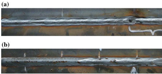
Fig. 2 Exemplary joint made with a corroded wire (S4), b contaminated with oil (S6)
