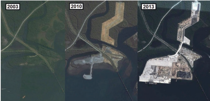
Fig. 11.2 Land reclamation in Santos estuary due to EMBRAPORT construction. (Source: adapted from Google Earth)
