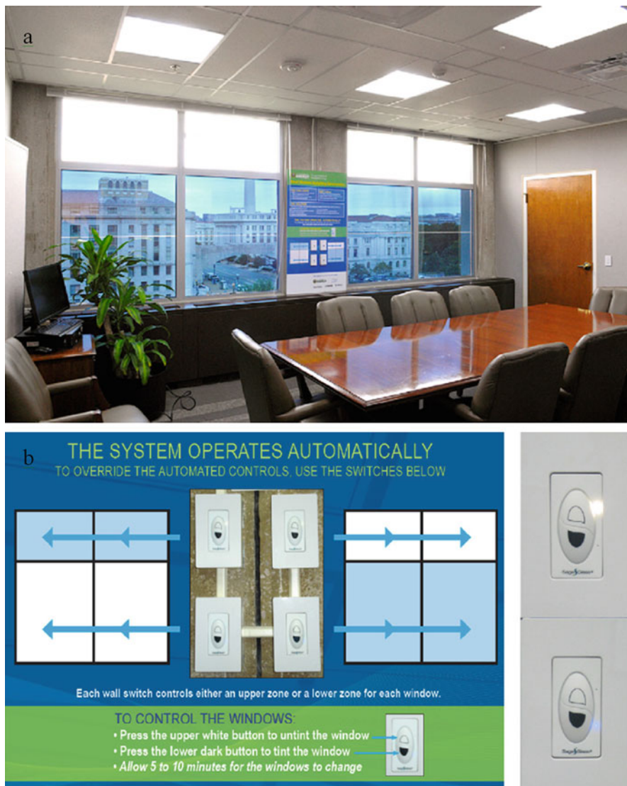
Fig. 18 (a) Interior view of the conference room with upper and lower control zones and (b) Signage instructing occupants on how to switch the windows. (Reprinted from Energy and Buildings, 47, E.S. Lee, E.S. Claybaugh, M. LaFrance, End user impacts of automated electrochromic windows in a pilot retrofit application, 267–284, Copyright (2012), with permission from Elsevier)
