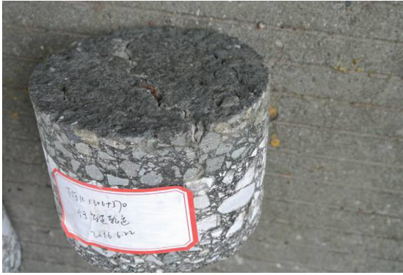
Fig. 1. Low-scaling transverse reflective crack
