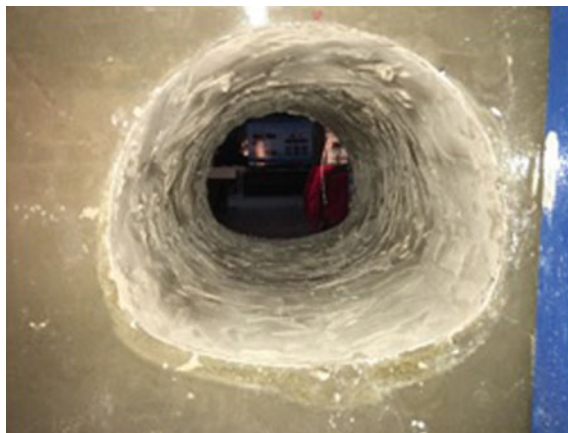
Fig. 11. Excavation of the third part of the tunnel
