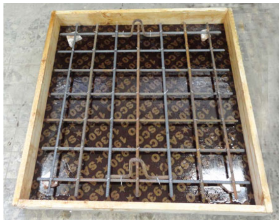
Fig. 2. Reinforcement and mold
