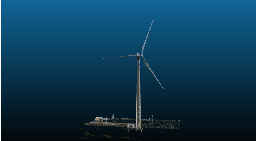
Fig. 2. The point clouds of the wind turbine collected by employing TLS.
