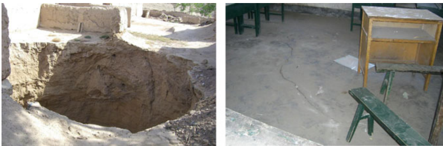
Fig. 1. Site condition of the ground above the coal mine
