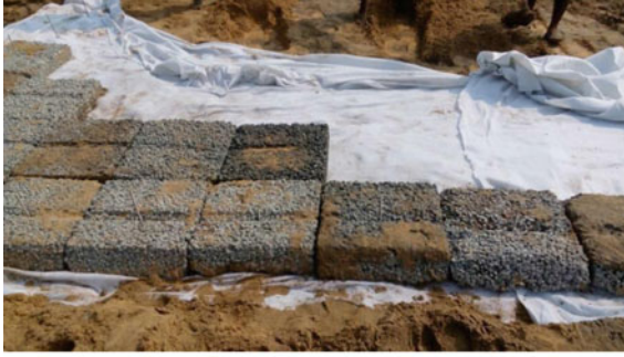
(a) Setup during installation
