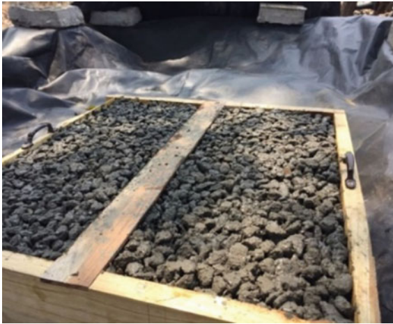
Fig. 4. Pervious concrete inside formwork
