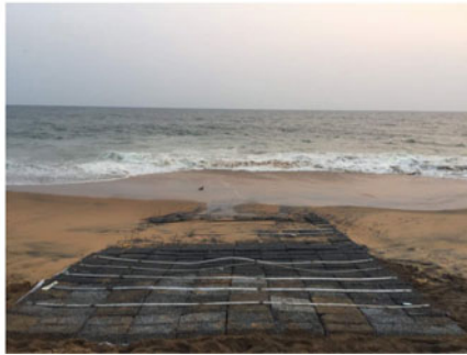
(b) Setup during installation
