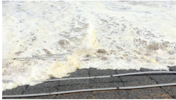
(a) Revetment exposed to frontal sea waves
