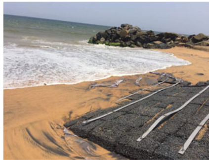
(b) Revetment exposed to frontal sea waves
