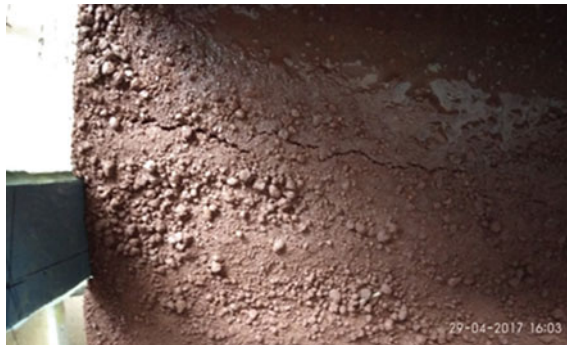
Fig. 25. Slope failure - 28° [soil - 3]
