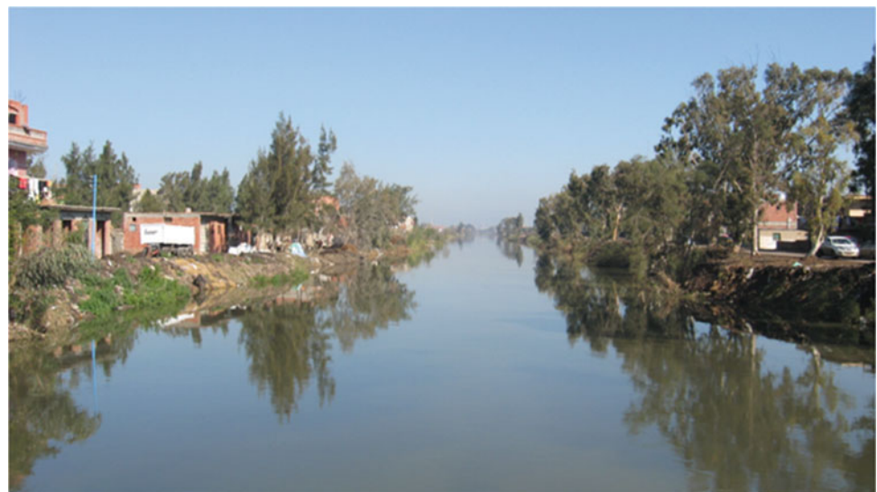
Fig. 1.6 The El-Gharbia drain (Kitchener) is one of the largest open drainage systems in the Nile Delta (about 59 km) and collects about 12% of the disposal water including agricultural and industrial effluents (from factories in Tanta, El-Mahalla El-Kubra, and Kafr El-Zayat to deliver into the Mediterranean Sea in Baltim and causes a pollution of soils around it). Photos by El-Ramady (2015)
