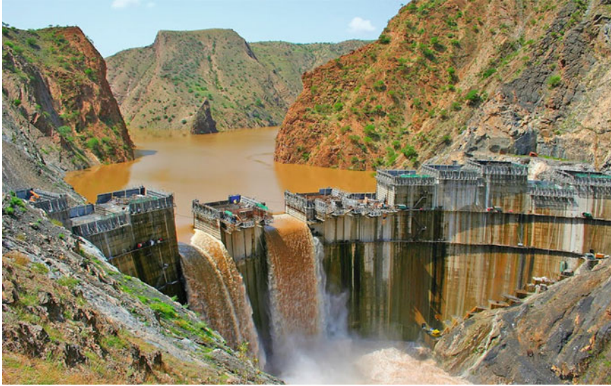
Fig. 9 Overtopping the Tekeze Dam due to large flood in September 2007 (Photographer Paul Snook: http://www.panoramio.com/photo/76171558 )
