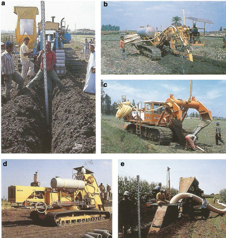
Fig. 7 Types of drainage machines used in Egypt [3]. (a) Concrete pipes (diameter 100 mm). (b) Corrugated PVC pipe (diameter 80 mm). (c) V-plough, trenchless drainage machine. (d) Concrete large-diameter pipes (150–400 mm). (e) Large-diameter corrugated PVC pipe (200–400 mm)
