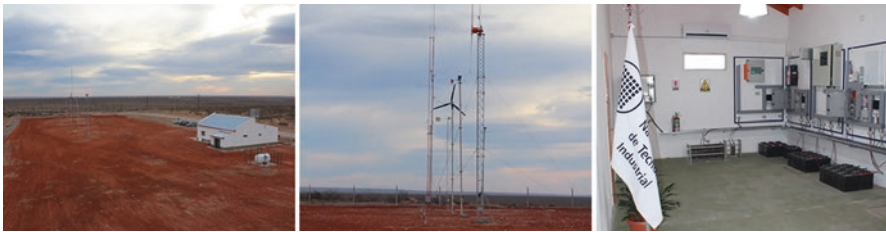
Fig. 4.6 INTI testing plant in Cutral C6, Neuquén [17]
