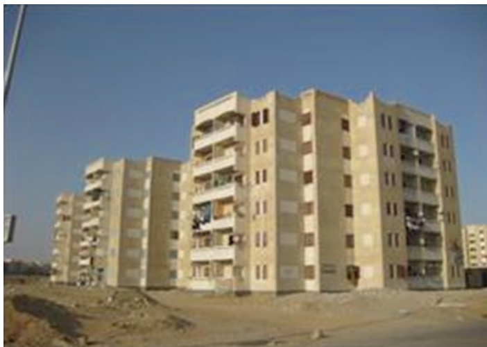
Fig. 2.1 Residential units for low-income class in 6th of October City, Egypt
