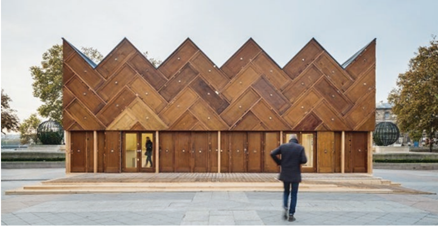
Fig. 31.2 Encore Heureux Circular Pavilion, Paris 2016. The temporary building was built with recycled products and subsequently dismantled with the complete recovery of material resources. (Photo by Cyros Corut courtesy of Encore Heureux Studio)
