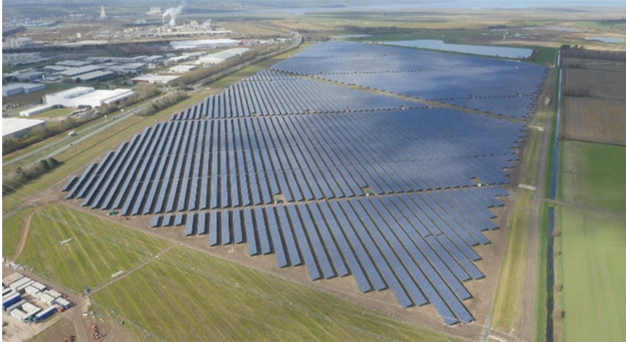
Fig. 36.4 The 50 MW Shotwick Solar Park on Deeside in North Wales
