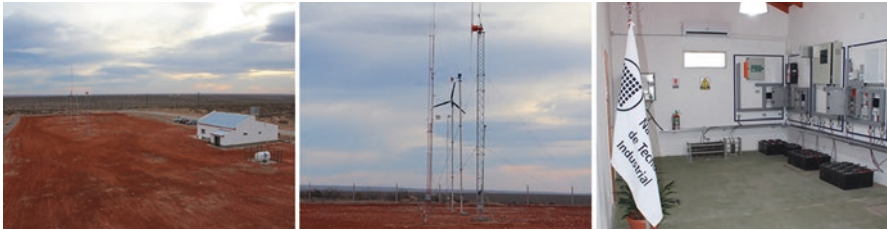
Fig. 4.6 INTI testing plant in Cutral C6, Neuquén [17]
