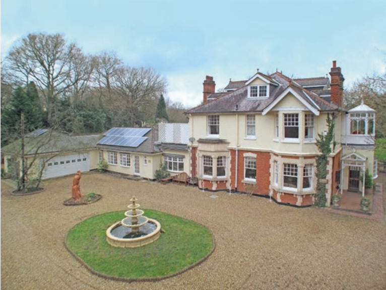
Fig. 36.1 A typical domestic installation of photovoltaic solar panels
