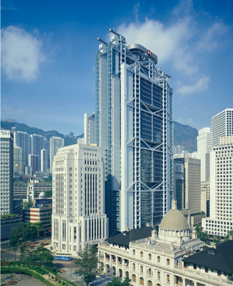
Fig. 31.4 Norman Foster, Hong Kong Bank, Hong Kong (RC) 1986. The project was designed to be dismantled into pieces, loaded on boats, and restored in another location (if China were to occupy Hong Kong)
