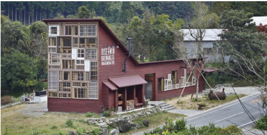
Fig. 31.1 Hiroshi Nakamura & NAP Kamikatz, Public House, Kamikatsu (J) 2016. The building was made of recycled and reused materials and products
