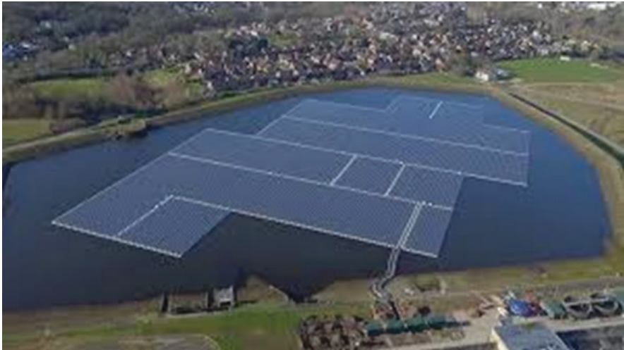
Fig. 36.3 Most solar pv capacity is now on the industrial scale. This is the 3 MW floating solar farm on Godley Reservoir, Tameside, Manchester, UK
