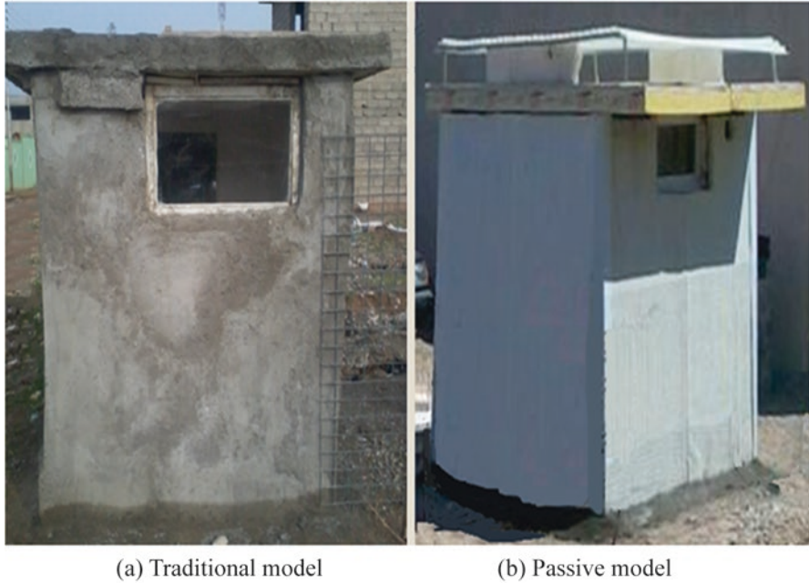
Fig. 21.2 Constructed models used in the study. (a) Traditional model. (b) Passive model
