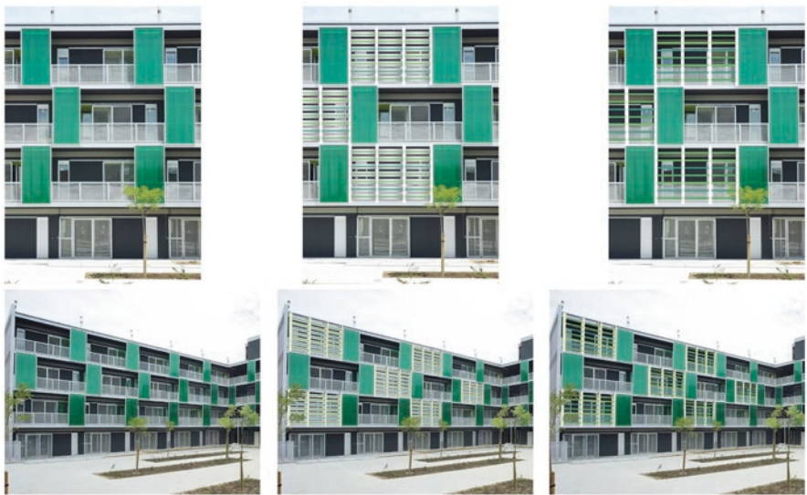
Fig. 28.5 Few photomontages of the integration of the solar concentrator in façade
