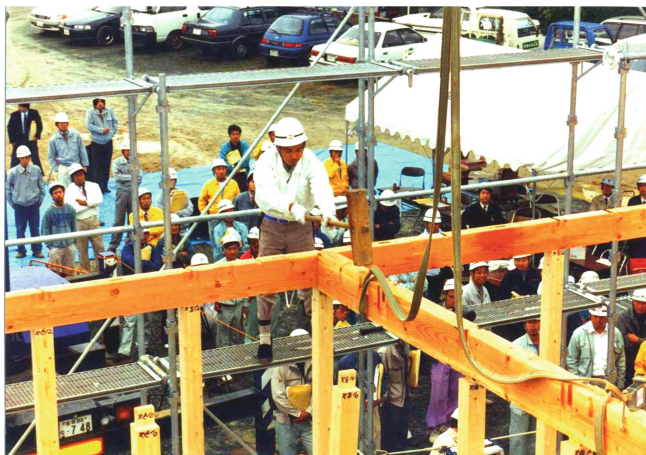
Fig. 5. Educating workers about the method at construction sites.
