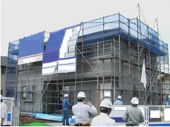
Fig. 4. A house constructed using this method.
