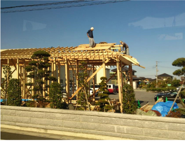
Fig. 2. Low-rise construction site from over thirty years ago.
