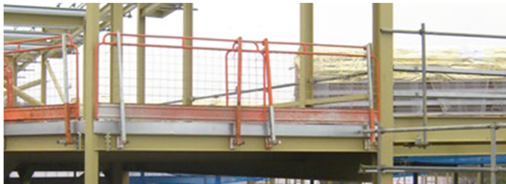
Fig. 5. Example of safety railing in a construction site.
