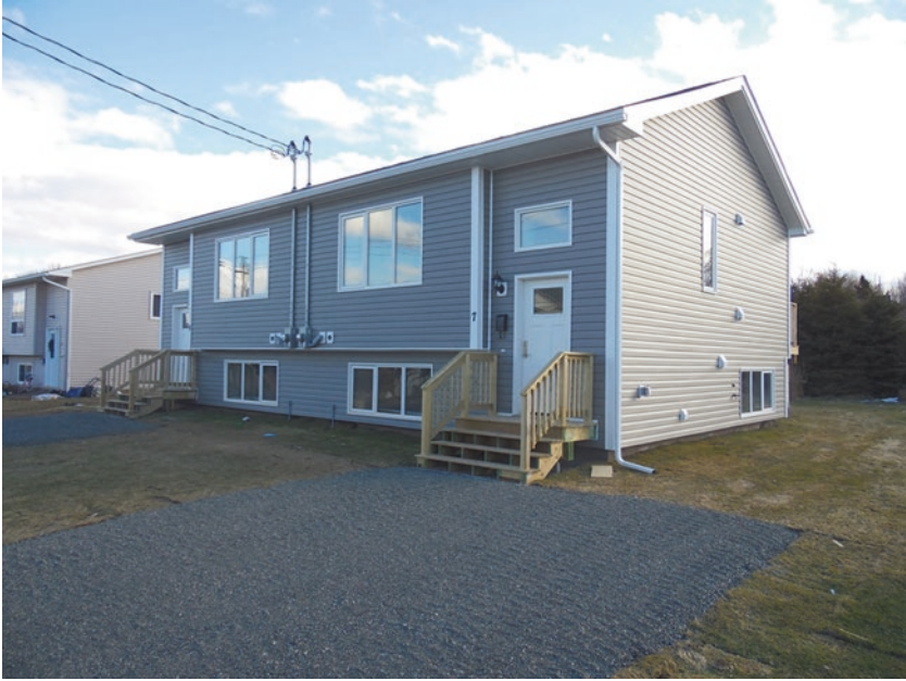
Picture 14.4 Amherst Passive House front view
