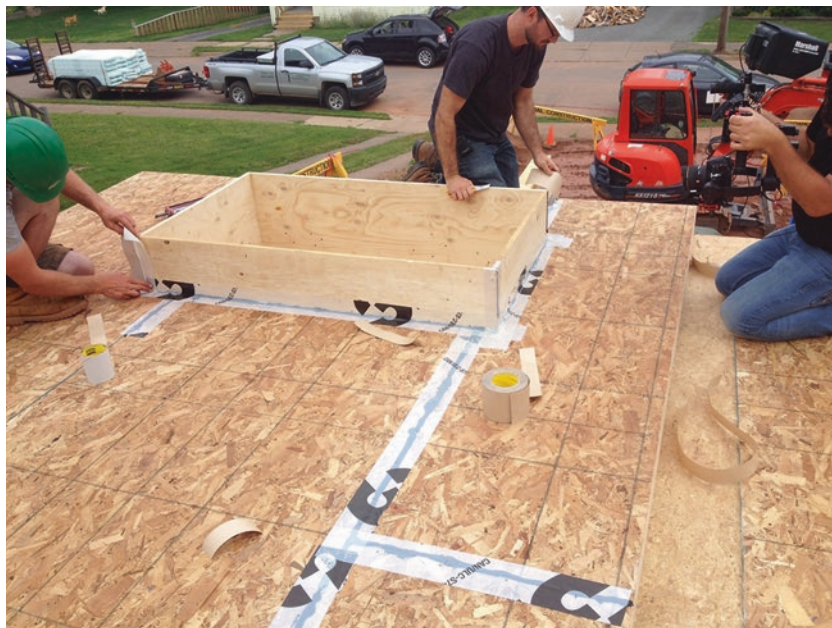
Picture 14.1 Truro Passive House video documenting air-sealing walls and penetrations
