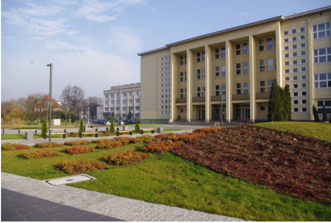
Fig. 1. Campus of the Silesian University of Technology after the revitalization. View of the building of the Civil Engineering Faculty and in the background visible is one of the laboratory buildings of the Chemistry Faculty. Photo taken by D. Winnicka-Jasłowska
