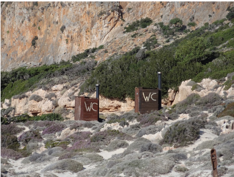
Fig. 2. Example of vault toilet, Balos Lagoon, Kissamos, Crete, Greece. (Source: own work)
