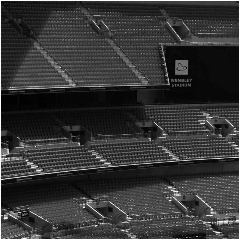
Fig. 7. The spectators communication and evacuation system applied to the tiers of Wembley Stadium . An example of classic vomitories with a gangways running tangent to their balustrades. Notice that the width of the vomitories has been decreasing on higher and higher tiers, while tier's capacity is growing; (Photo: M. Pelczarski)
