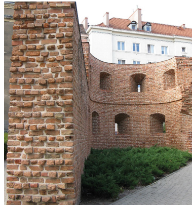
Fig. 2. Poznan, Gunpowder Tower, embrasures inside of the wall (author)
