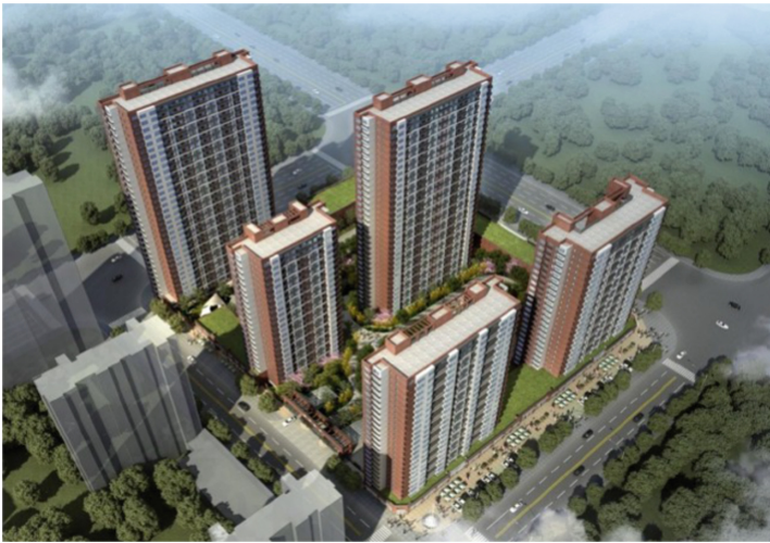
Fig. 1. Shandong Binhe new home public rental housing project. Bird view (author: Xiaolei Wang).
