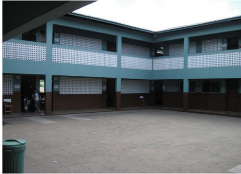
Fig. 2. Patio from the municipal Governador Moura Cavalcanti school. Source: original
