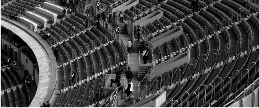
Fig. 6. The vomitories and gangways system on the Stadium Slaski eastern stands - aerial view. The upper tiers' stairs were moved to the middle of the rows between the vomitories; the level of the first row of this tier has been significantly raised, improving the field of view of spectators occupying these places; (Photo: author)
