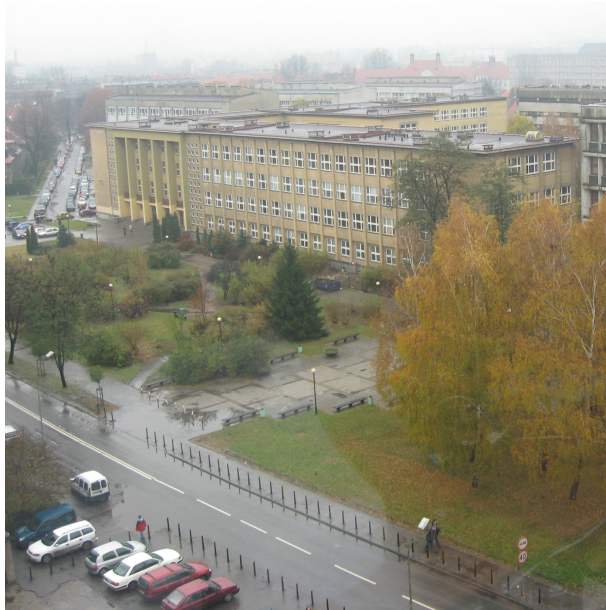
Fig. 1. The view in the direction of the main space of the campus of the Silesian University of Technology - as of November 2009; in the foreground one can see the Akademicka Street, in the background the edifice of the Faculty of Civil Engineering is visible (photo taken by Joanna Tymkiewicz)
