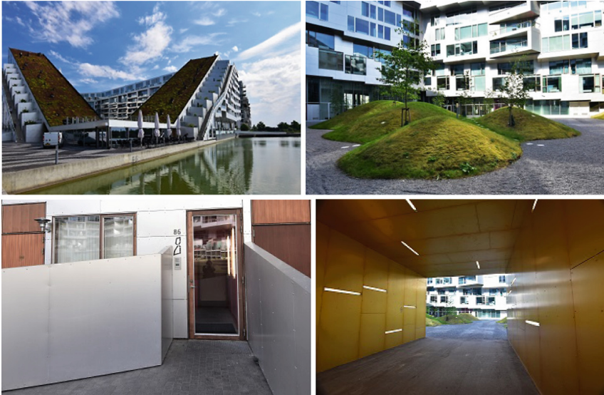
Fig. 2. Multifamily building in Copenhagen in Ørestad, Denmark, 8 HOUSE, Bjarke Ingels Group (BIG) archives project from 2010. (photo A. Gumińska, 2016)
