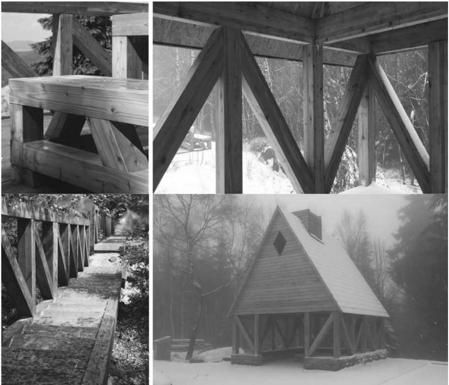
Fig. 9. A building details, shelter in winter [3]. Maciejko A, Strzelecki M.: Design of a small technical infrastructure of the Stołowe Mountains National Park, Strzelecki Biuro Architektoniczne, [3].
