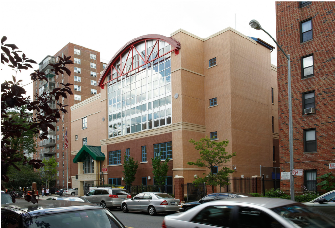
Fig. 5. Front elevation of PS 244Q- The Active Learning Elementary School. Four floors primary school surrounded by much higher residential towers. Distinguished main entrance feature at the right scale. phot. A. Dudzinski
