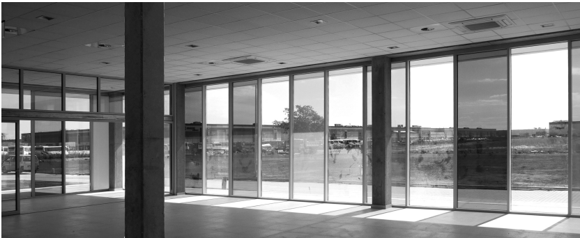
Fig. 2. 3D printing factory, design Horn Architects. Canteen with kitchenette in the office building and common spaces serve the whole of staff including production, managing and IT employees. Windows have colorful “spacer” panes, fully visible depending on the daylight or internal lighting, canteen is connected with outdoor terrace. There are also conference and meeting facilities and lunch rooms. Photo by the author.
