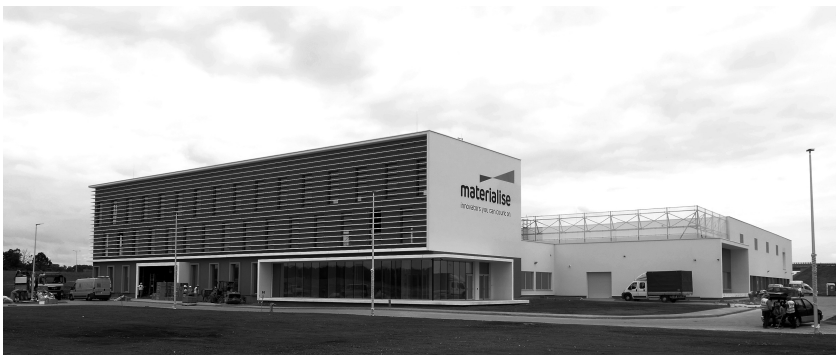
Fig. 1. 3D printing factory for Materialise, design Horn Architects. On the left – office building with canteen for all staff, on the right – production building with scanning unit and technical roof behind aluminum mesh screen. Both buildings are joined by a connecting space of communication/lounge with green wall and the sculptural, 3D printed tree. The article was written in the final period of construction of the factory (2016–2017). Photo: finish of construction, July 2017. Photograph by the author.
