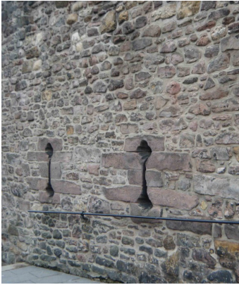
Fig. 1. Edinburgh Castle, outside slits of embrasures, shaped for archer and musket fire (author)
