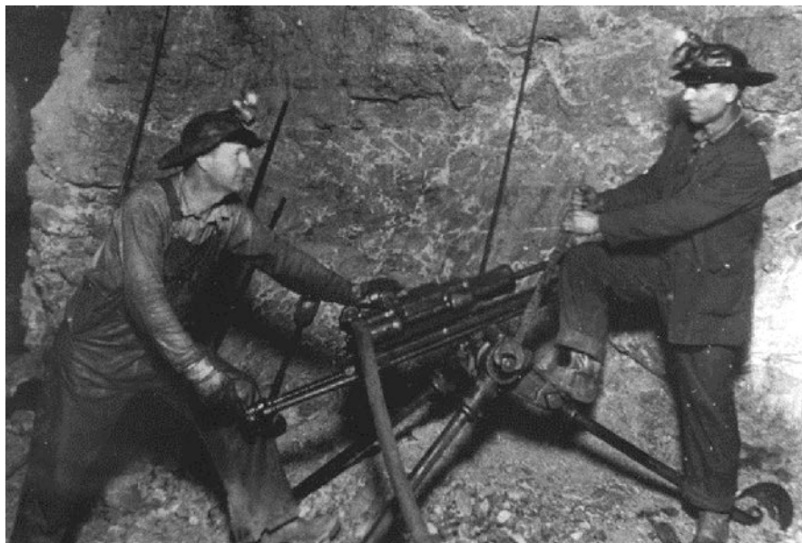
Fig. 3.5 Rock drills driven by compressed air replaced hand-jacking for drilling shot holes, here in an underground mine
