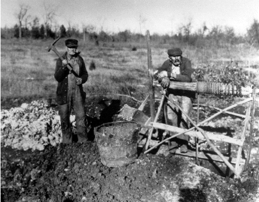
Fig. 3.1 Exploring for ore circa 1880. Ore samples are being extracted from a test shaft in the Tri-State lead-zinc district (Missouri, Kansas, Oklahoma)
