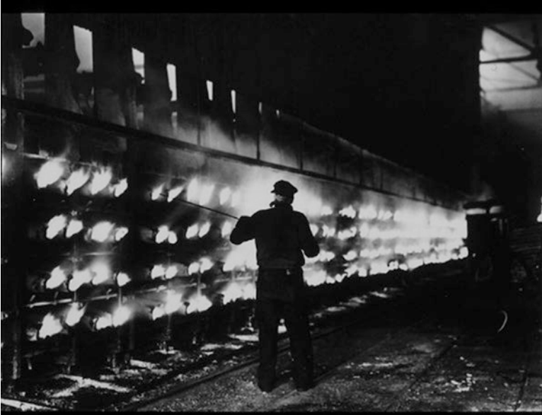
Fig. 3.17 In the Belgian retort furnace, zinc ore is reduced to metal vapor that is collected in condensers. The residual carbon monoxide reducing gas burns at the condenser mouths
