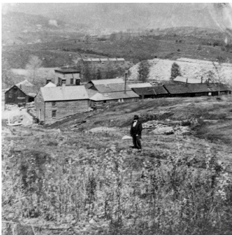
Fig. 3.8 Mowbray built his blasting-oil works at the western end of the Hoosac tunnel adjacent to its spoil piles, seen here in the background of the picture. (Mowbray photograph)
