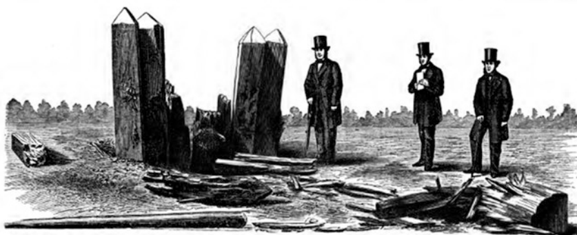
Palisade after the explosion of a 25-lb. box of gun-cotton. From a photograph.
