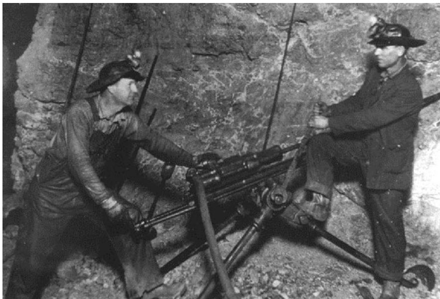
Fig. 3.5 Rock drills driven by compressed air replaced hand-jacking for drilling shot holes, here in an underground mine
