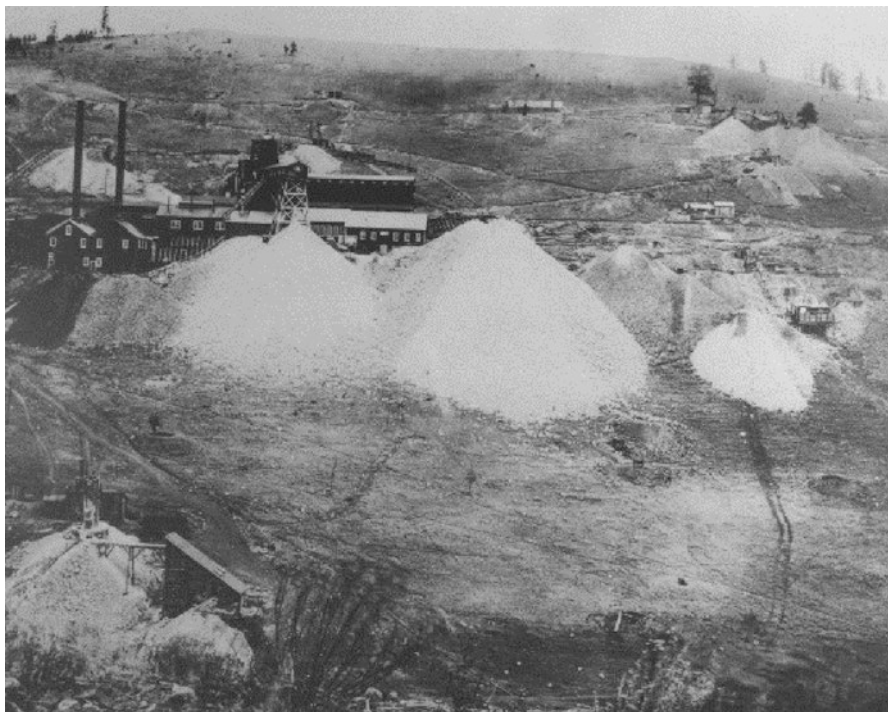
Fig. 3.3 Milling circa 1880. Stamp mills in Colorado discharged ever-increasing wastes without recovering much metal. What became of them was someone else's problem
