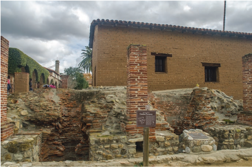
Fig. 4.8 Remains of a Catalan forge at Mission San Juan Capistrano, CA. These bloomery furnaces were built in 1797 and supplied wrought iron for making tools at the mission. These are the oldest metalworking structures in California. (Photograph by W. Hsieh, 2015, used under Creative Commons License Non-Commercial 2.0. www.flickr.com/photos/whsieh78/24266319841/ )
