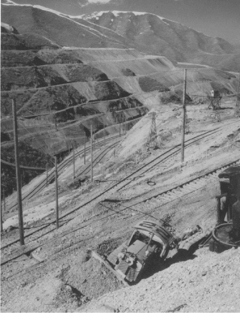
Fig. 3.7 Miners at the Bingham pit in Utah took out ore on rail cars running on tracks laid on benches built on the steep sides of the excavation
