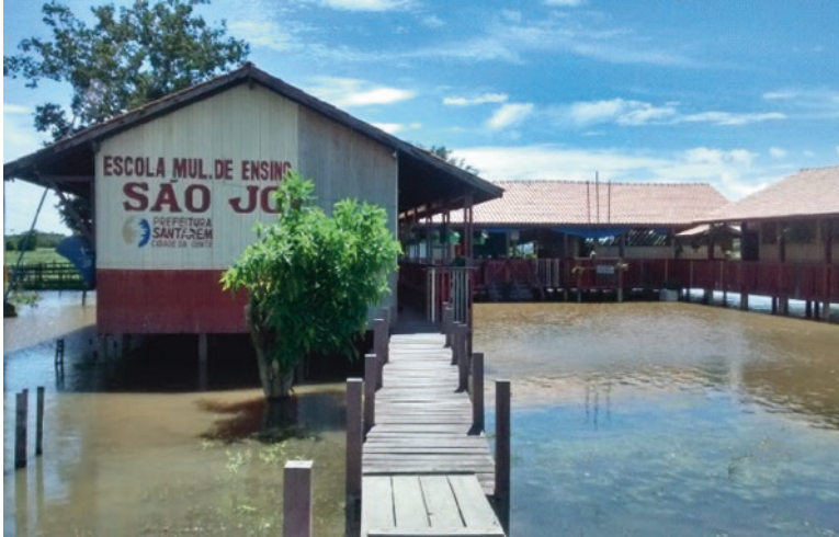
Fig. 3.1 São Jorge County School, Tapará Grande. (Source: The author (April/2015))
