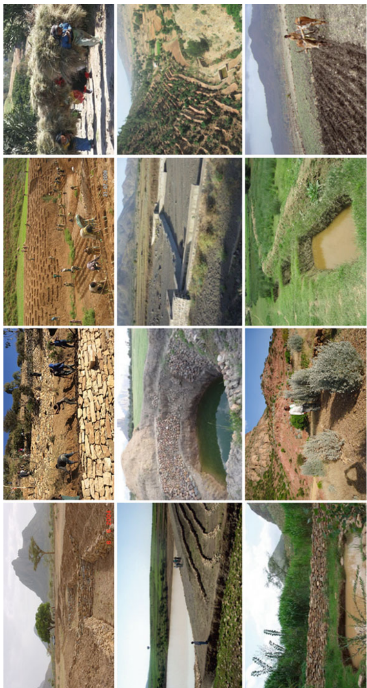
Fig. 4 Different EBA interventions implemented in Tigray (Top row right to left: Gully treatment, stone bunds, integrated gully treatment, zero-grazing (cut and carry from exclosures). Middle row: Reservoirs, hand-dug wells, and river diversion). Bottom row: Treated gully, enclosure enriched with drought-tolerant halophytes, earth sided deep trenches, the derbero system of plowing)
