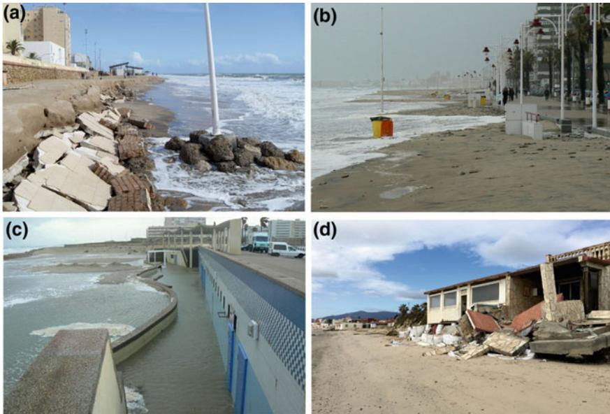
**Fig. 14.6** Examples of storm impacts at urban beaches along Cadiz coast. **a** Damage to coastal protections at La Victoria beach (Cadiz) in April 2015. **b** Seafront overtopping by storm surge at La Victoria beach (Cadiz) in January 2010. Note that dry beach width in this area is commonly 40 m. **c** Flooding of beach facilities at Cortadura beach (Cadiz) in March 2010. **d** Damage to seafront house at El Rinconcillo beach (Algeciras) in March 2017
