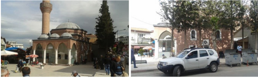
Fig. 8.1 General appearance of the Mosque
