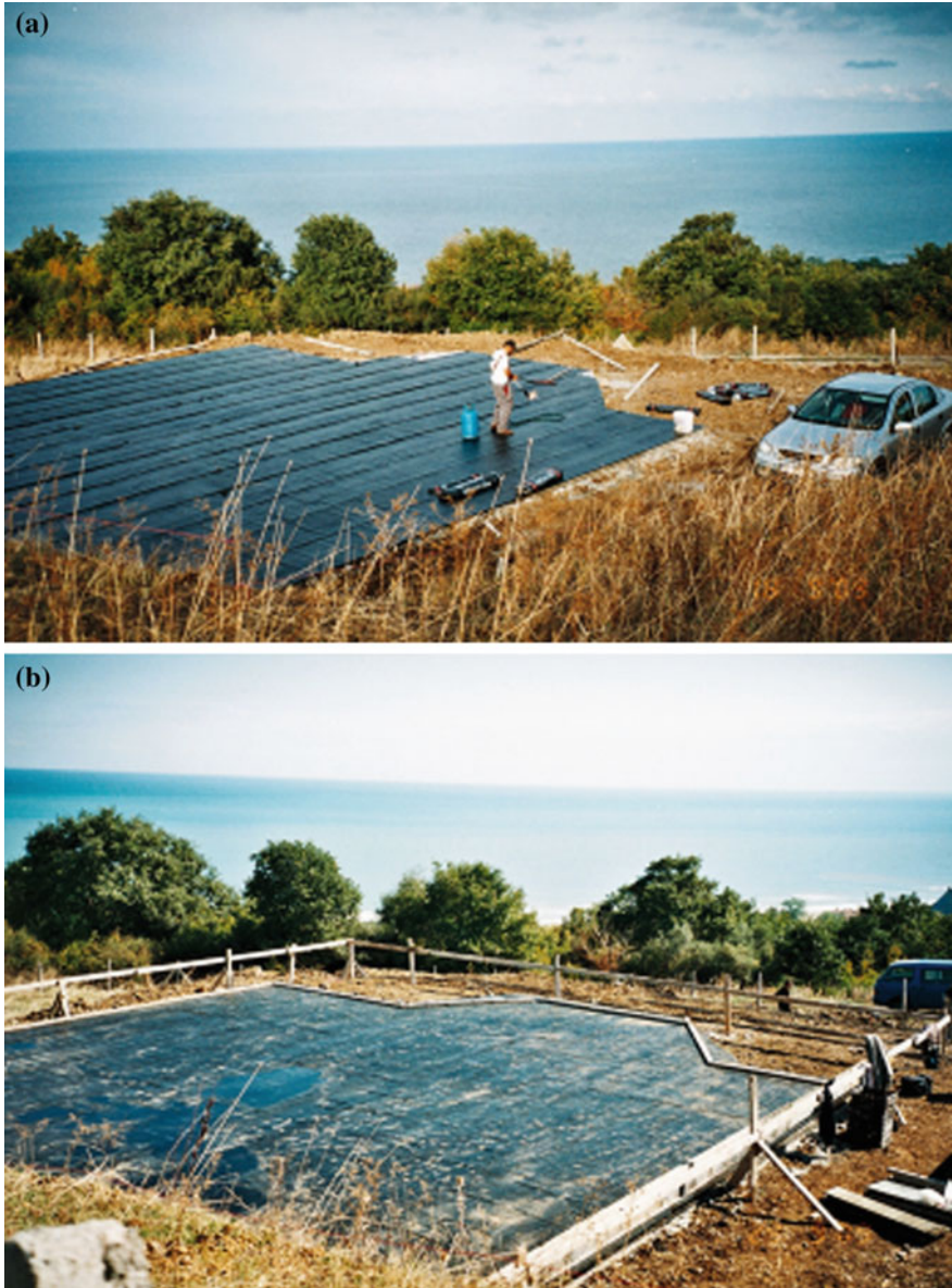
Fig. 3.5 First natural seismic isolated (NSI) private building in Turkey/Samsun (Incesu Mah. Sirincak Sok. No: 2/1) a Preparation of the friction interface—Level 1 b Preparation of the friction interface—Level 2 c General view of building—SN direction d General view of building—NS direction
