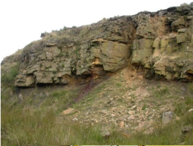
Fig. 7 Mass failure in overlying sandstone due to removal of mudstone support
