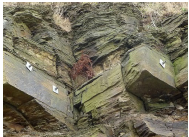
Fig. 13 Spot treatment with pre-stressed rock nails for reinforcement of individual blocks
