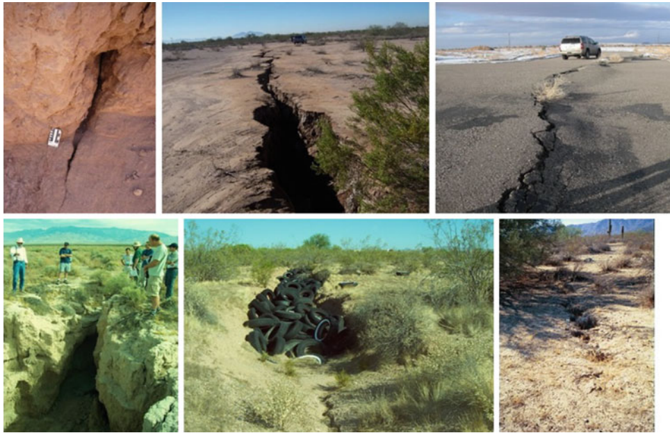
Fig. 1 Examples of earth fissures. Beginning clockwise from the top left: (1) un-eroded incipient earth fissure in bottom of trench excavation at powerline FRS in Central, Arizona, (2) fresh earth fissure gully at Siphon Draw Wash Basin in Central Arizona, (3) earth fissure with
