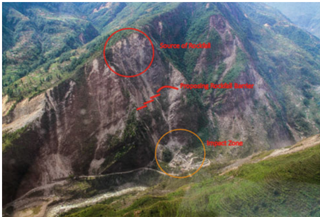
Fig. 3 Rockfall problem in Upper Bhotekoshi Hydropower Project after the Gorkha Earthquake
