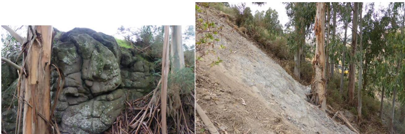
Fig. 7 Discrete rockfall source before (left) and after (right) removal of source
