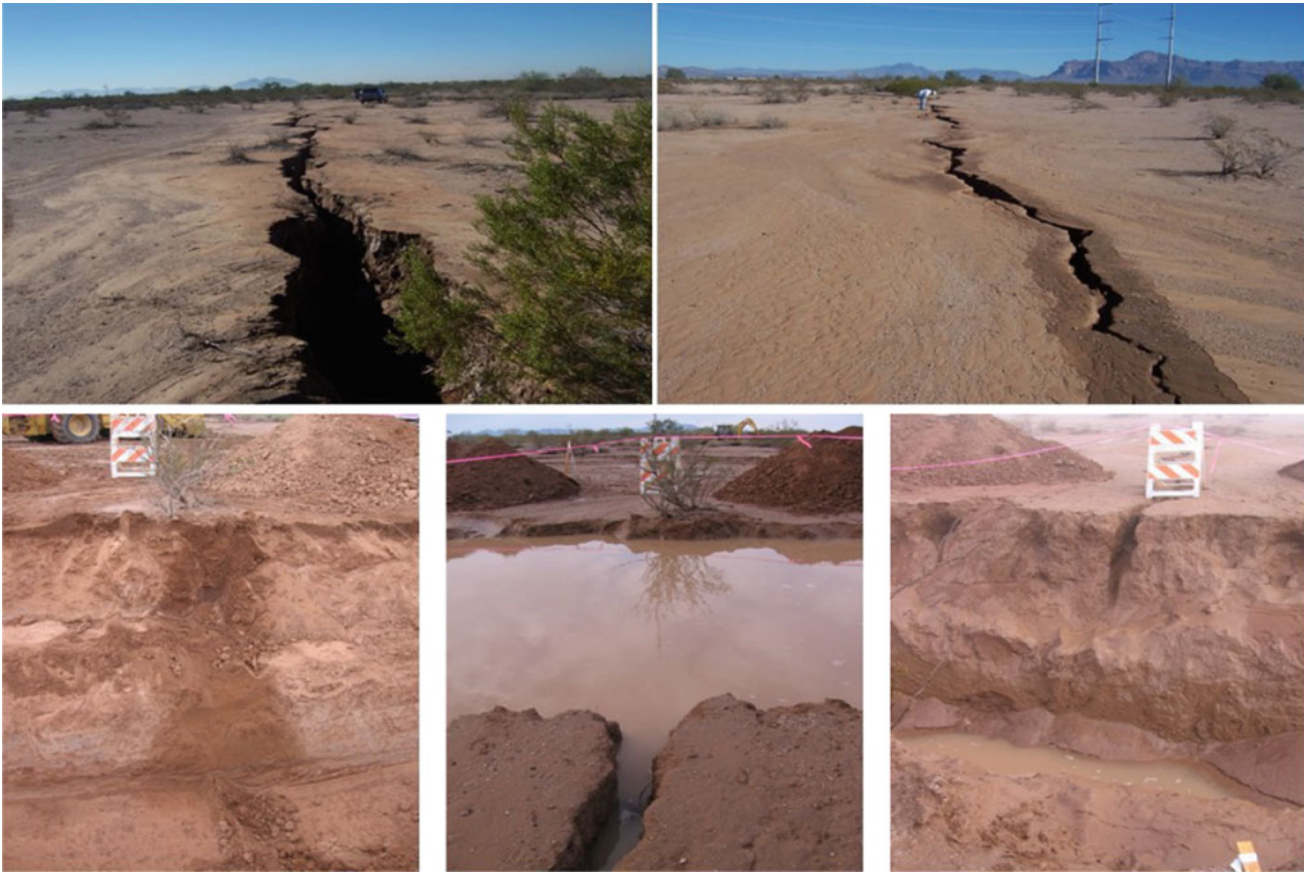
Fig. 2 View of the SWEF prior to construction of the SDW Detention Basin. The upper 2 images show the extension of the earth fissure that occurred overnight as the result of a rain event. The bottom three photos show the trench at the termination of the SWEF. The left image shows
