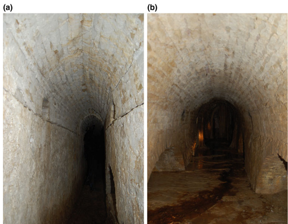
Fig. 6 a The drainage system: branch B. b Vertical shaft in the branch B
