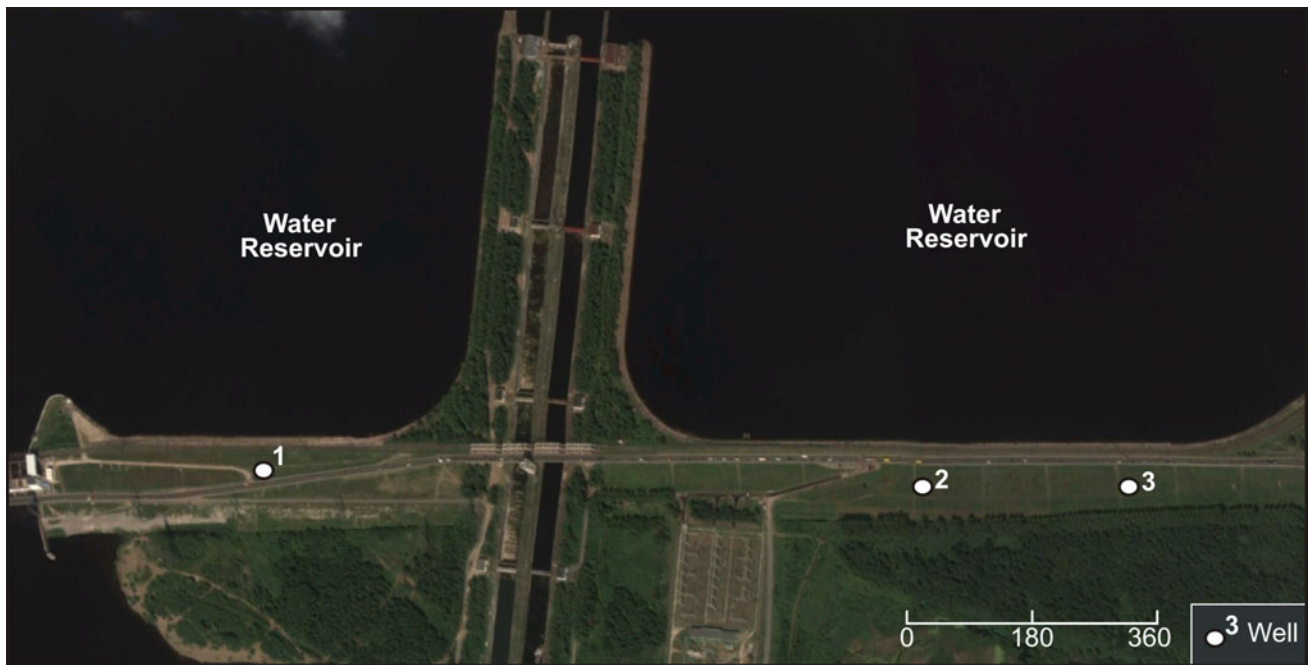
Fig. 2 Location of wells in the dam
