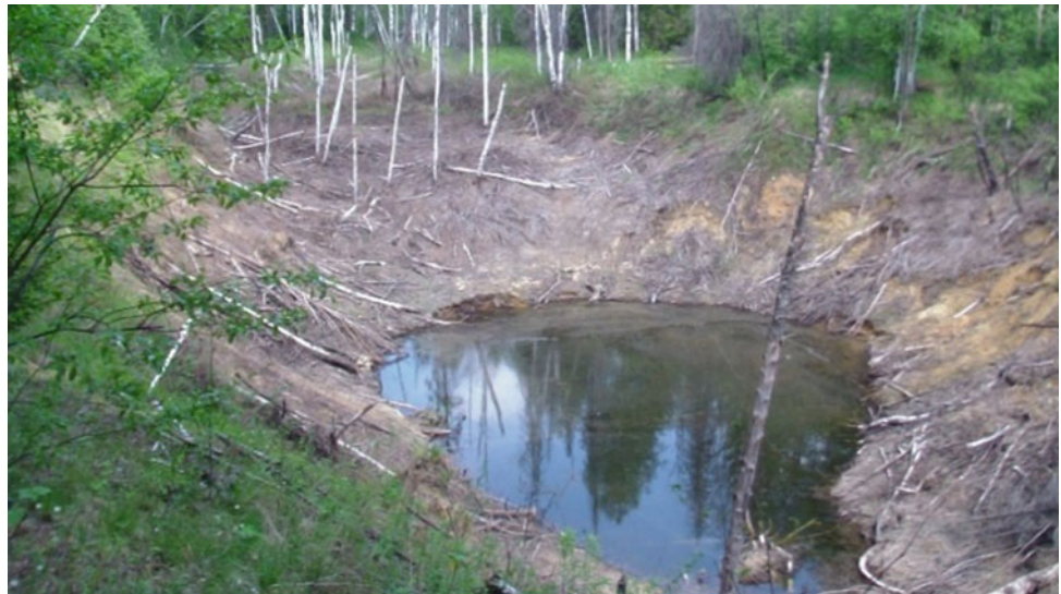
Fig. 5 Failure over the mine field of the Krylatovsky mine, Sverdlovsk region
