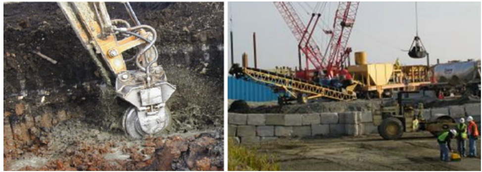
Fig. 2 Left photo: excavator mounted soil mixer, Right photo: Pugmill mixing
