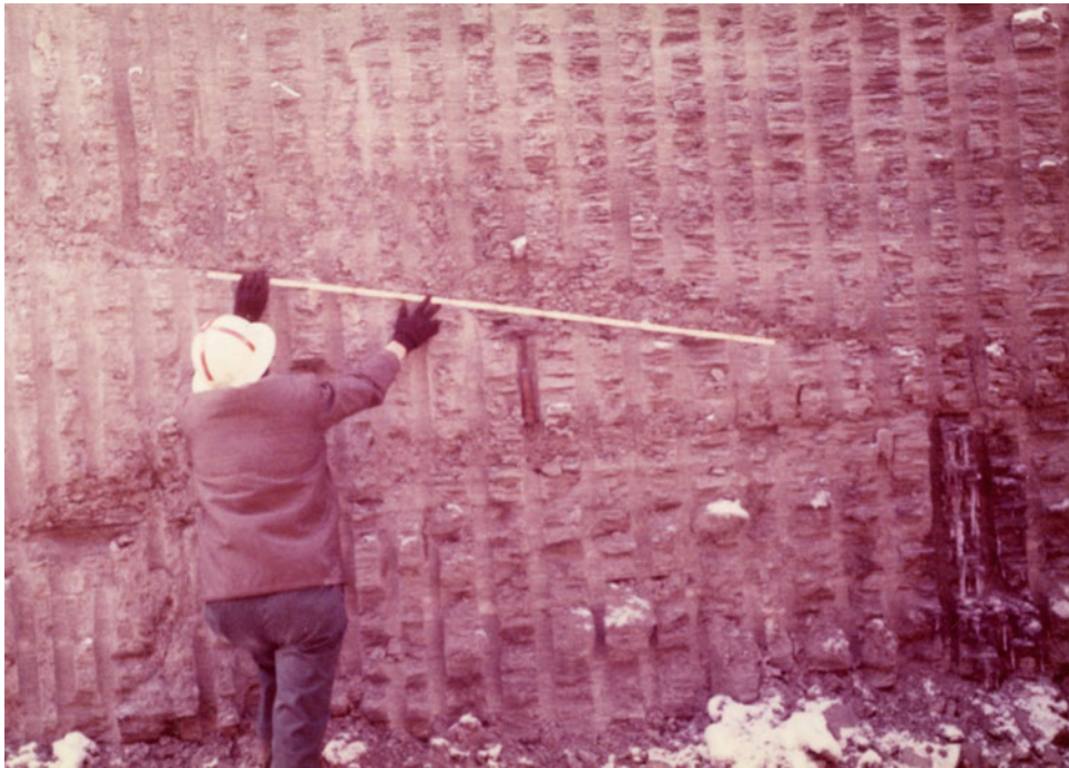
Fig. 2 Thrust Fault in Dam Foundation Excavation, early 1960s (photo by Harry Ferguson)
