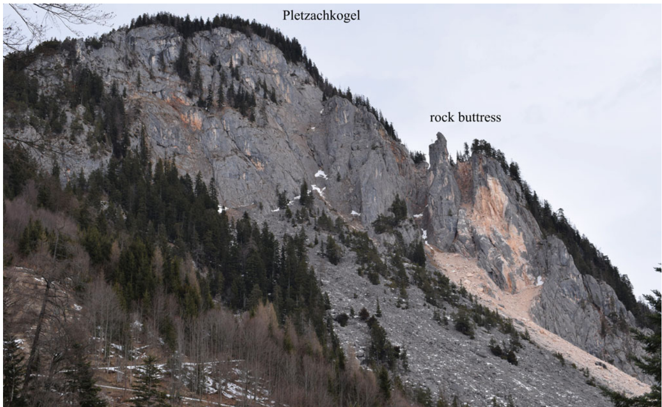
Fig. 2 The southeastern cliff face of the Pletzachkogel (left) and the rock buttress (right). The source areas and deposits of the 2011 and 2015 rock falls are indicated by freshly exposed rocks in the buttress area. Note major joints shaping the rock mass
