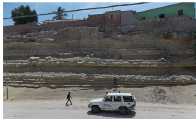
Fig. 2 Slope 4, with intercalated layers of limestone and marls
