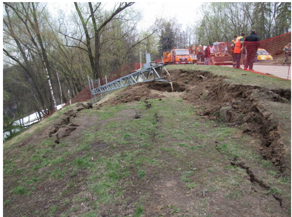
Fig. 9 Place of landslide activation in Vorobyovy gory
