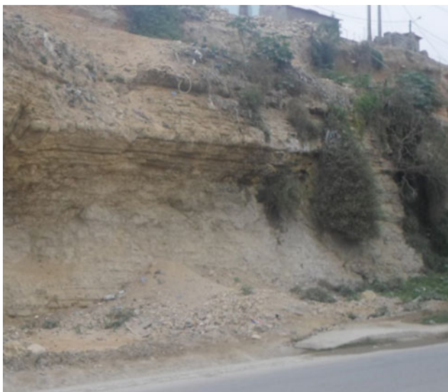
Fig. 1 Slope 1, erosional features leading to rockfalls
