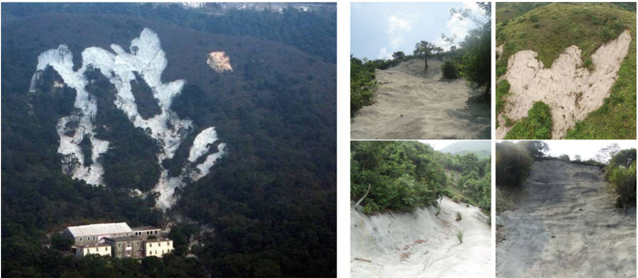
Fig. 2 Site condition following the implementation of urgent repair works
