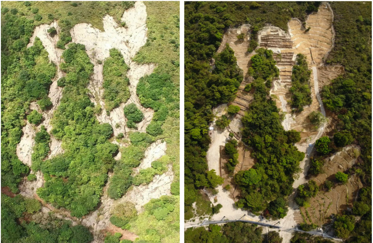
Fig. 6 Pre- and post-construction site conditions
