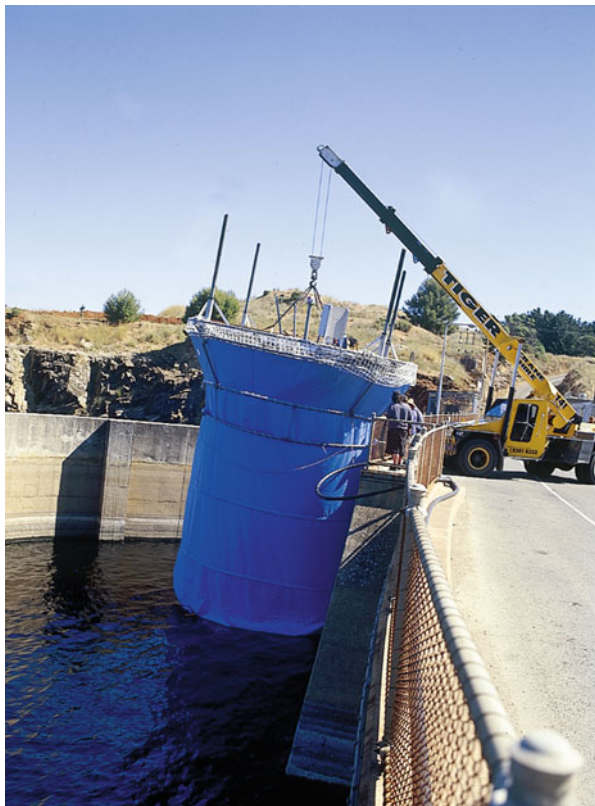
Fig. 6.4 A surface mounted mixer being deployed in Myponga Reservoir in South Australia
