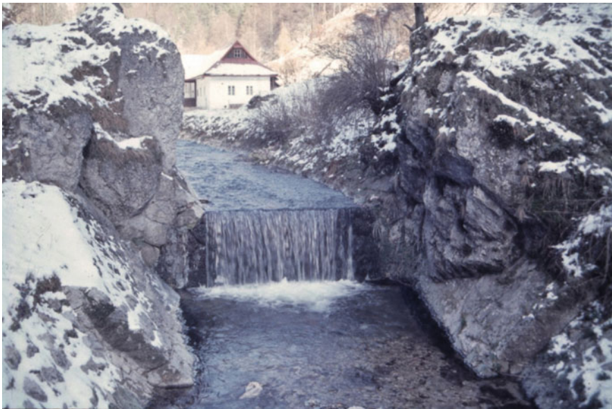
Fig. 4 The weir built in natural rock of oldest torrent control in Hornojelenecká Valley from 1926 to 1927 and the torrent Jelenec in Slovakia (photo M. Jakubis)
