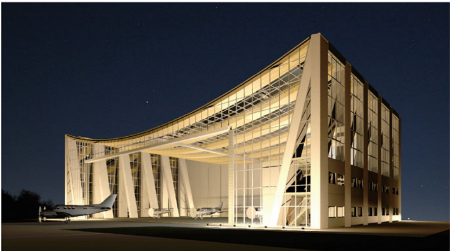
Fig. 2.1 A 3D model serves as the basis for a rendering to create a photo-realistic impression of a building design. (© C. Preidel, reprinted with permission)
