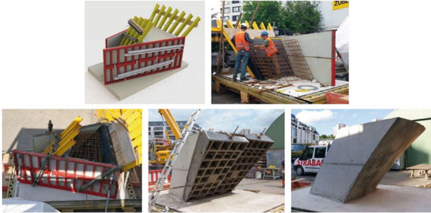
Fig. 26.22 Design-to-production process for a parabolic concrete column segment. (Strabag 2016, reprinted with permission)
