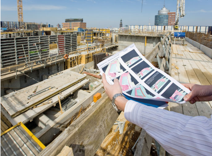
Fig. 30.7 Comparison of 4D model with actual status. (© HOCHTIEF ViCon, reprinted with permission)
