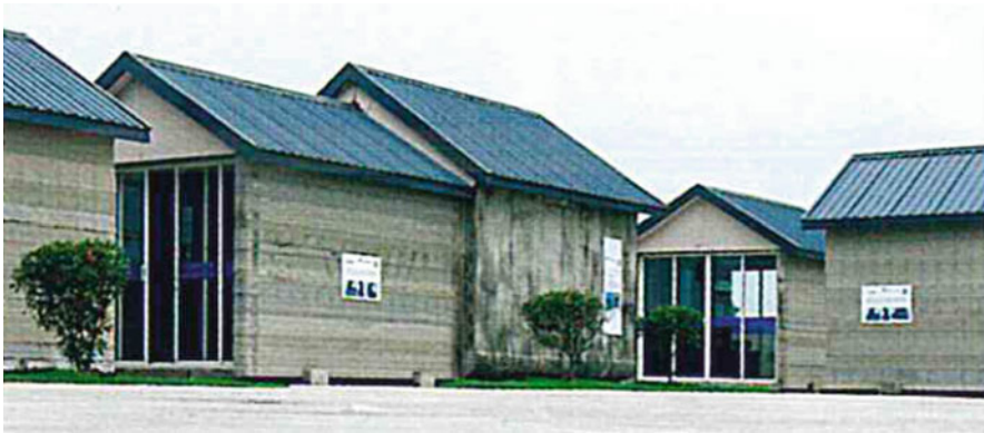
Fig. 26.8 House assembled from printed basic elements, manufactured by Winsun. (© Voxeljet AG, reprinted with permission)
