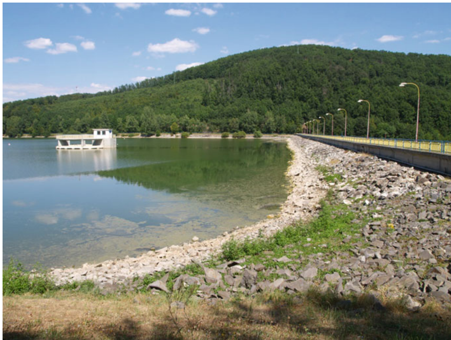
Fig. 2 Dam for irrigation water Ružiná (Photo: Jurík 2014)
