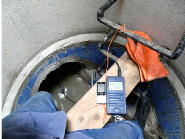
Fig. 13 Measuring device in a manhole
