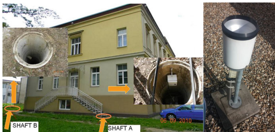
Fig. 7 Infiltration shafts located near building PK6 and rain gauge located on the roof of the University library
