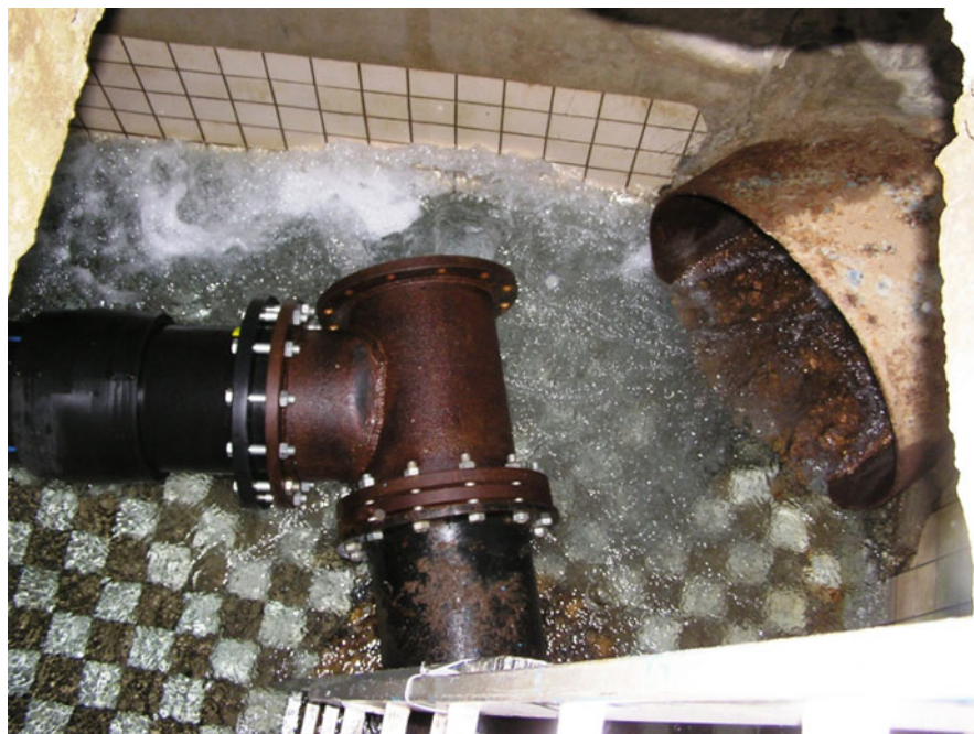
Fig. 21 Artificial lowering of groundwater head by pumping of groundwater excess to the Neresnica brook (Photo: M. Fendeková)
